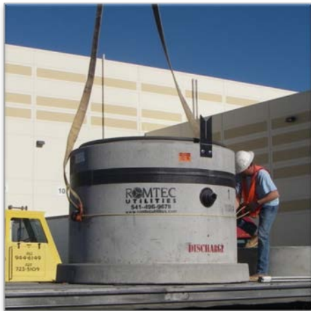
Figure 3: Using Romtec Utilities Uplift Brackets
