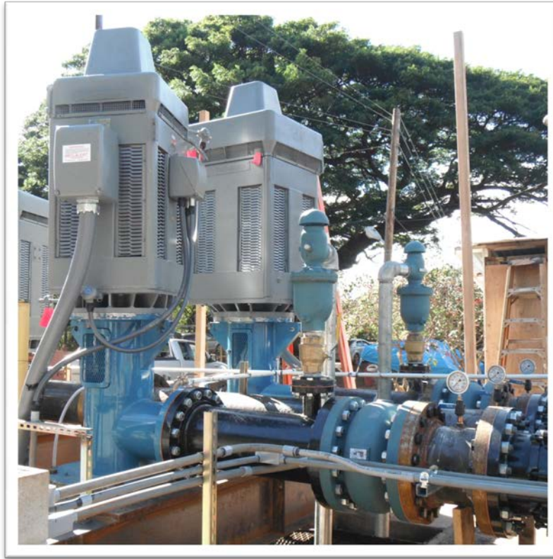
Figure 1: Triplex 450 hp Turbine Pumps & 12-Inch ID Above-Grade Valve Assembly
