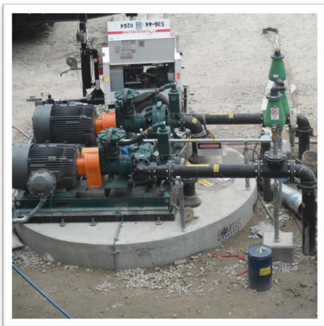
Figure 2: Above-Grade Discharge with Vacuum Assisted Self-Priming Pumps
